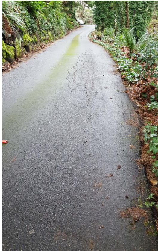
Plate 2. View of the upper (mid-west) section of private street, approximately looking west.
