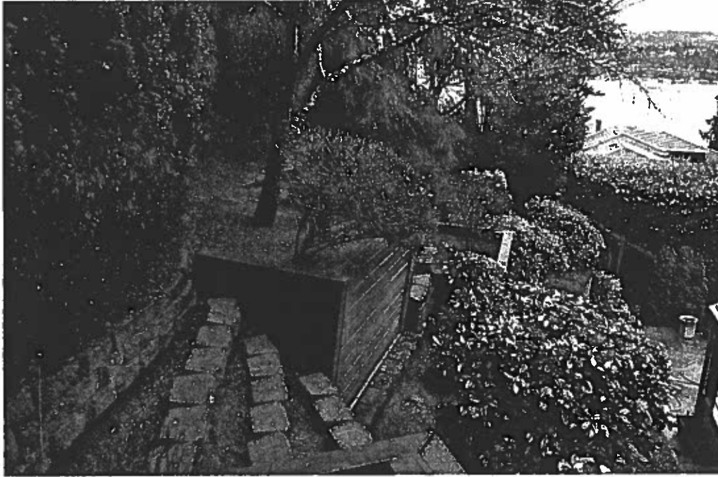
11. Retaining walls supporting access road between hairpin turns.
