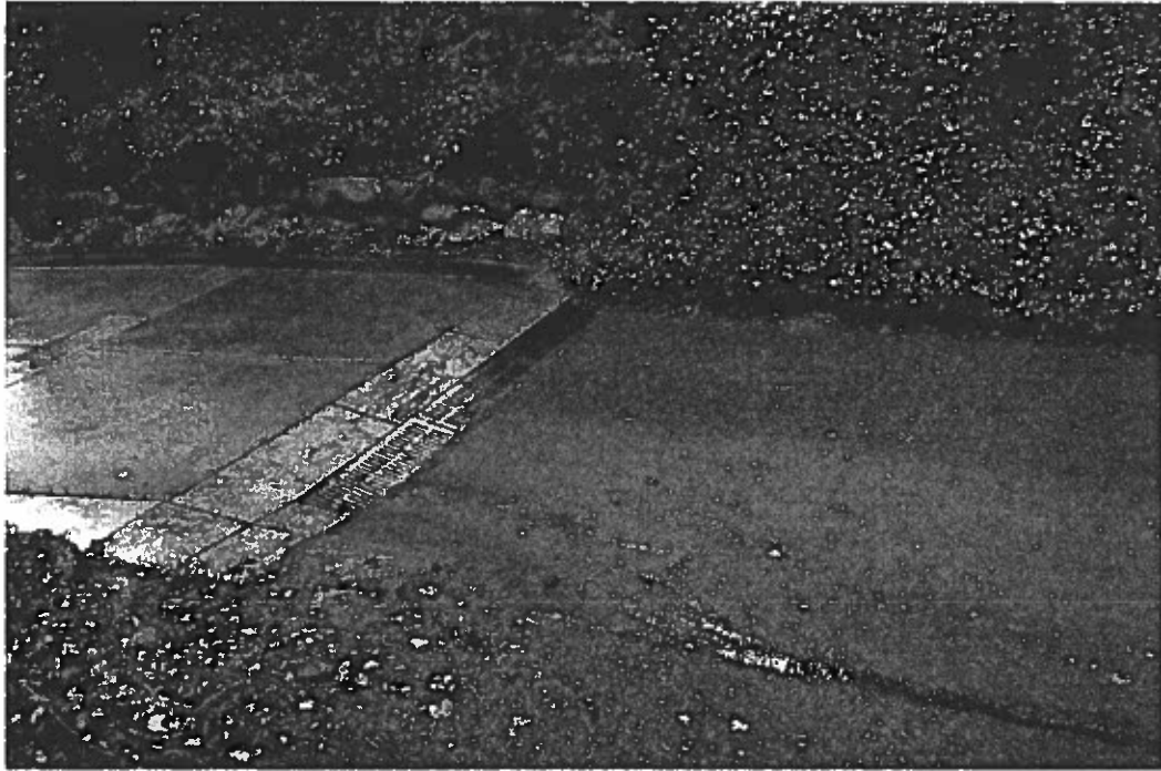
13. Trench drain at east end of access road.
